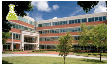
200 WEST STREET WALTHAM
