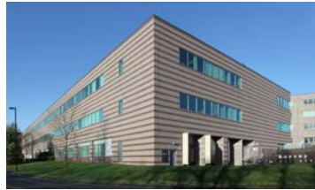
250 CAMPUS DRIVE MARLBOROUGH
