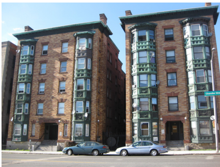
VENDOME & ST. IVES APTS WORCESTER 44 UNITS
