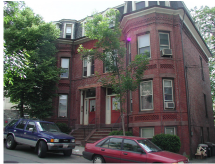
54-82 MT. VERNON ST SOMERVILLE 23 UNITS
