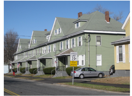
115-133 GRANT STREET FRAMINGHAM 22 UNITS
