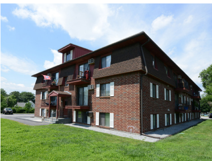
VALLEY GROVE APTS MANCHESTER, NH 95 UNITS
