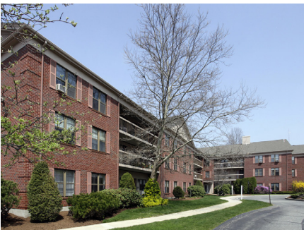
WEBSTER GREEN APARTMENTS NEEDHAM 76 UNITS
