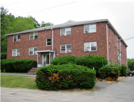
PARK AVE WEST 330 NESMITH STREET LOWELL 67 UNITS
