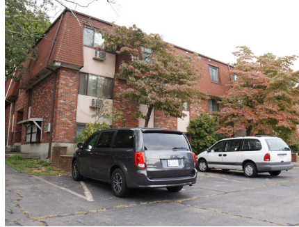
LIBRARY APARTMENTS NORTH ATTLEBORO 41 UNITS
