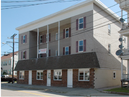
166-174 PINE STREET NORTH ATTLEBORO 20 UNITS
