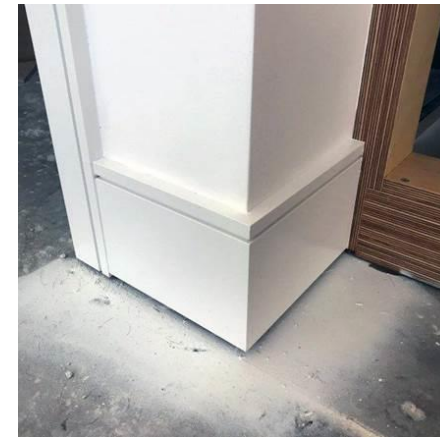
Painted base moulding and door casing detail
